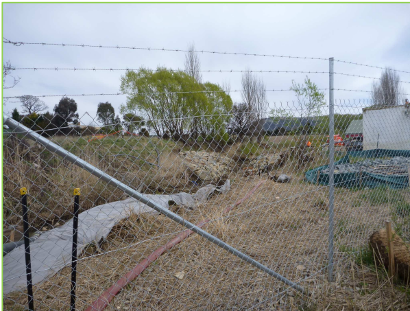
Plate 2. Looking just upstream of Williamsdale Bridge
