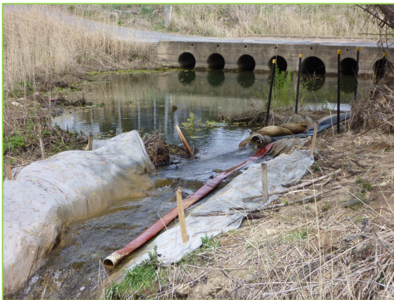
Plate 3. Creek water diverted to the downstream section of Burra Creek (left) and silt boom in place downstream of hose discharge
