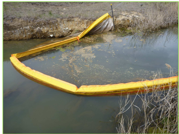
Plate 3. Creek water diverted to the downstream section of Burra Creek (left) and silt boom in place downstream of hose discharge
