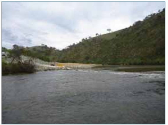
MUR 19. Looking across the riffle habitat towards the M2G intake structure
