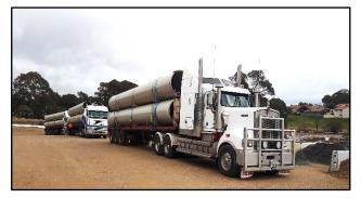
1.8m sewer pipes arriving to the primary compound by truck ready for unloading and installing
