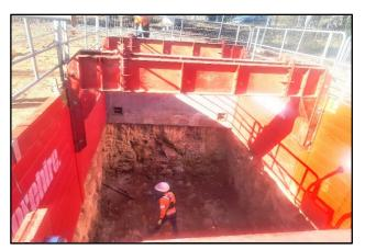
The launch pit dug out and ready for the microtunneling machine to start underboring
