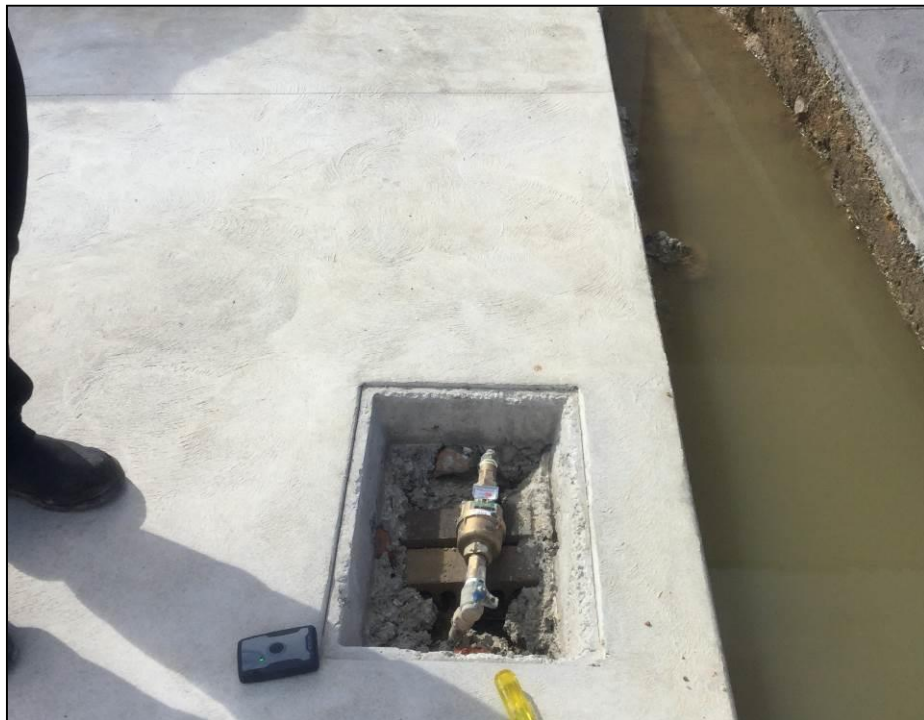
Fig. 10.4 Failed DN20 Water Meter Installation (Water meter in driveway and meter too high)
