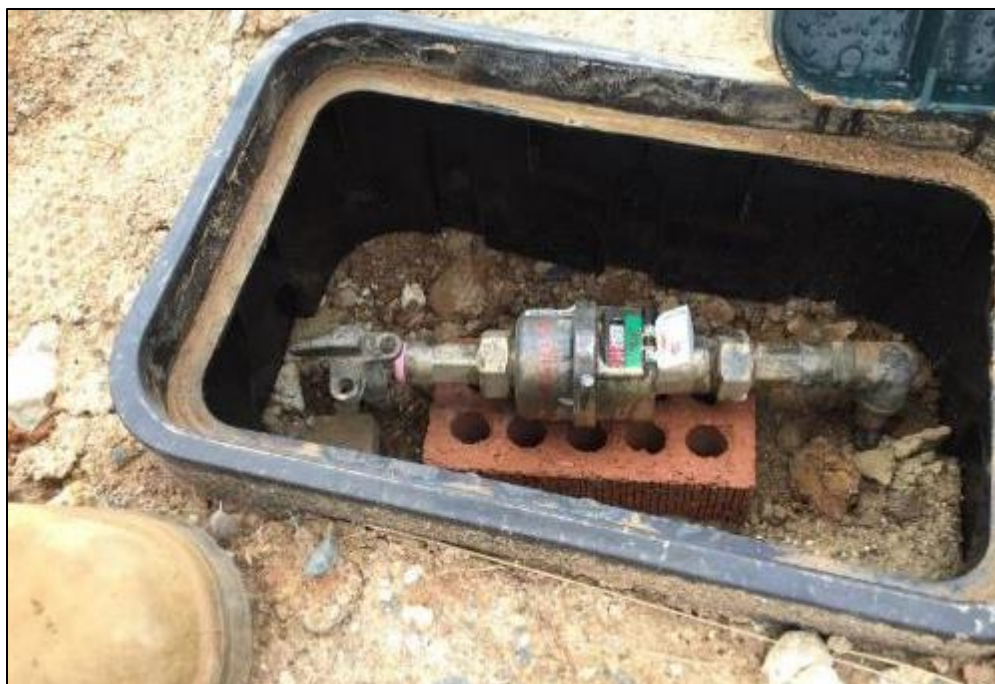
Fig. 10.1 Failed DN20 Water Meter Installation (Not centred; PE100 riser downstream)
