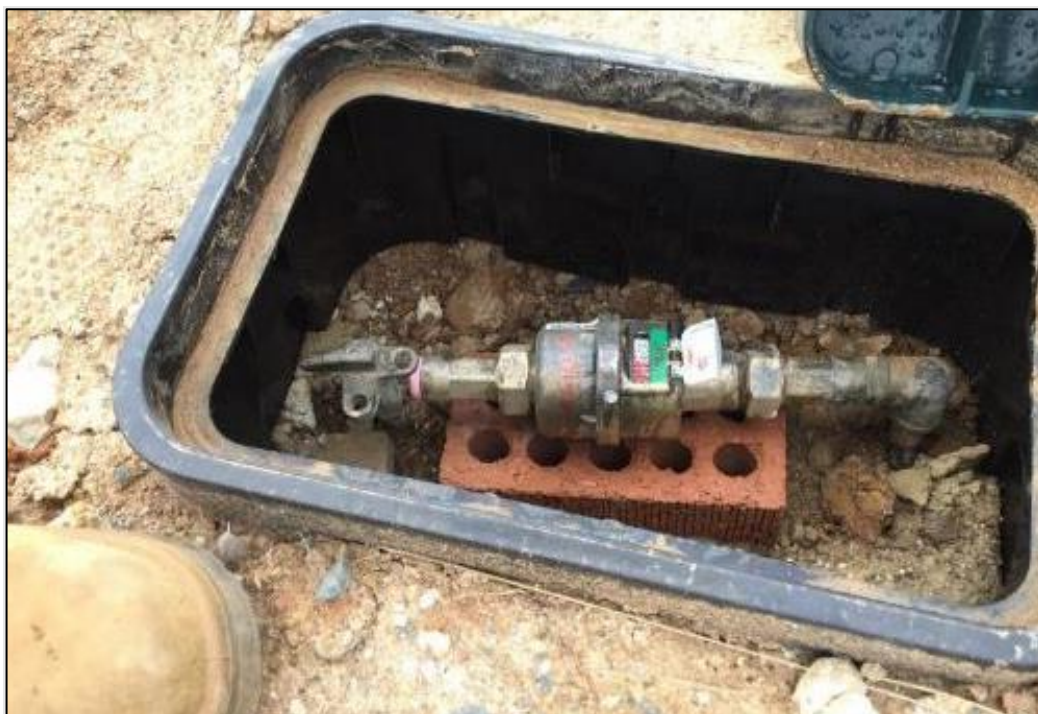
Figure Appendix A1 Failed DN20 Water Meter Installation (not centred; PE100 riser downstream)
