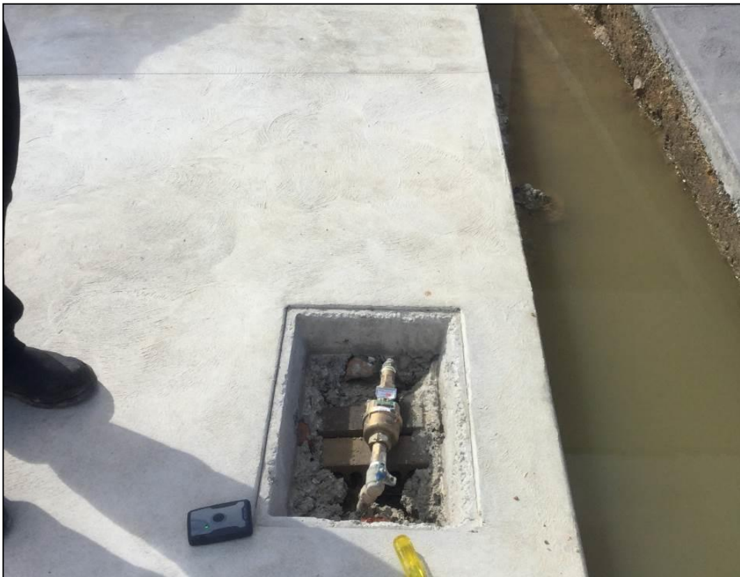
Figure Appendix A4 Failed DN20 Water Meter Installation (water meter in driveway and meter too high)
