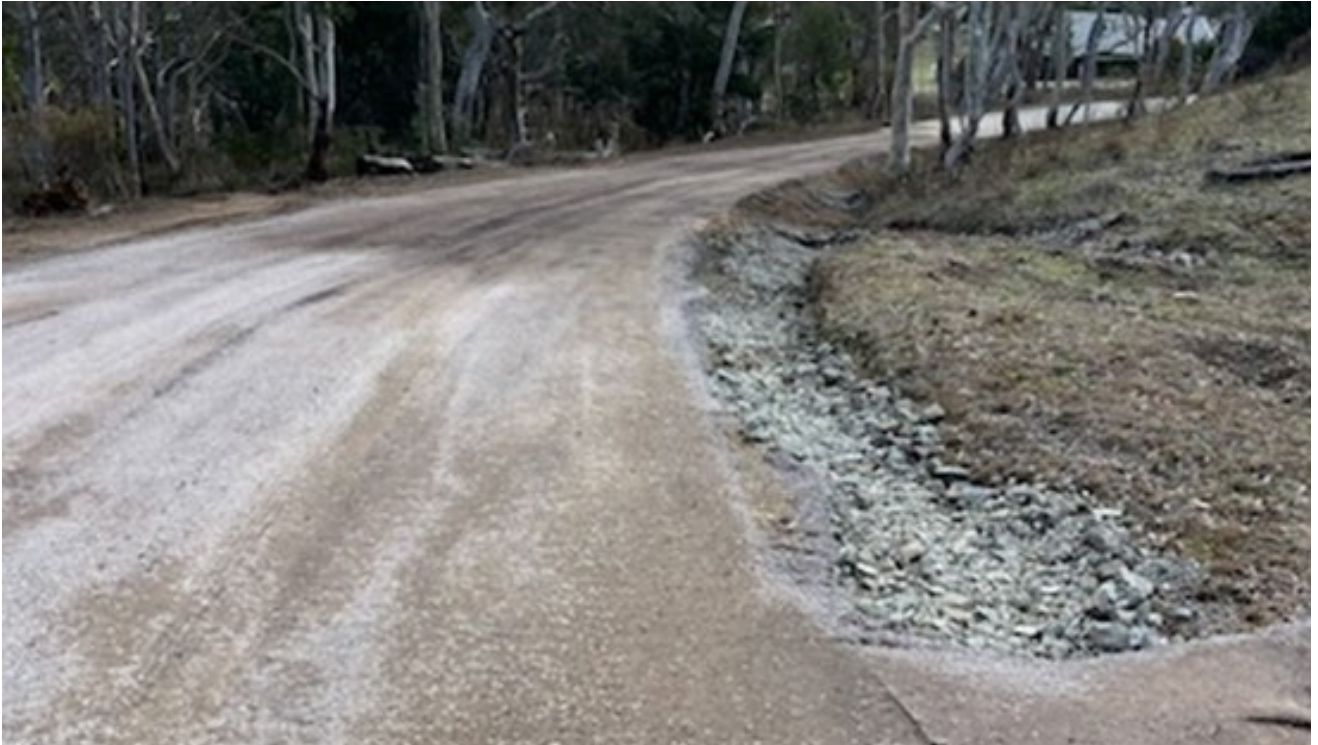
Gungahlin Reservoir Access Track and Drainage Repairs
