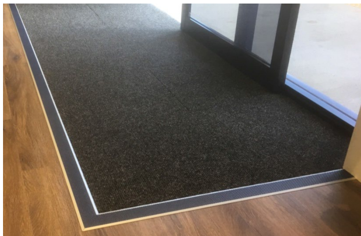
Figure 2.13.3 Edge bevelling of a surface differential (i.e. floor mat) in a door way
