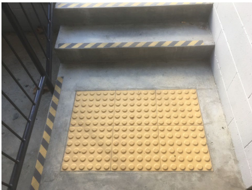
Figure 2.13.1 Proprietary anti-slip tiles embedded within a stairway landing
