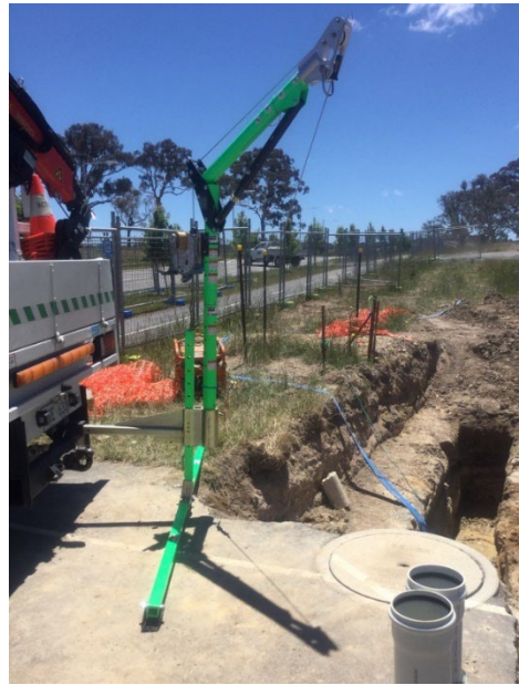
Figure 2.7.2 A tow-bar mounted davit being set-up over a maintenance hole
