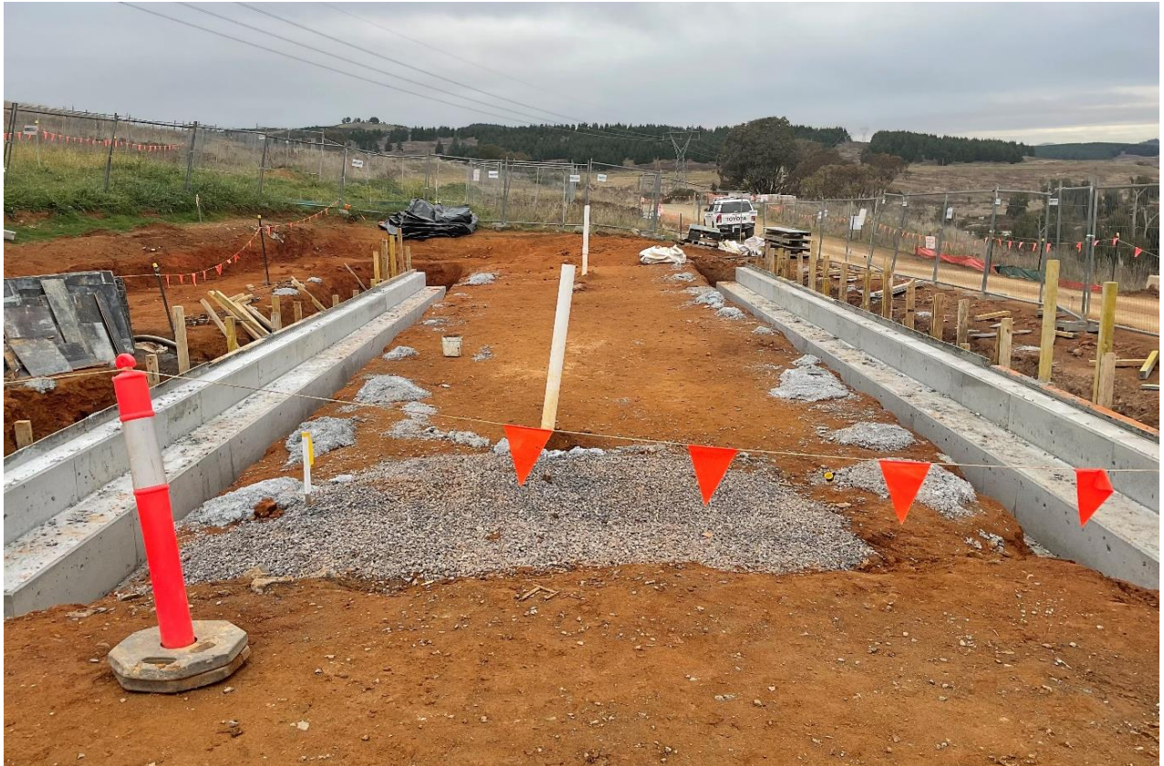
Figure 5.8.7 Bridging slab (under construction)
