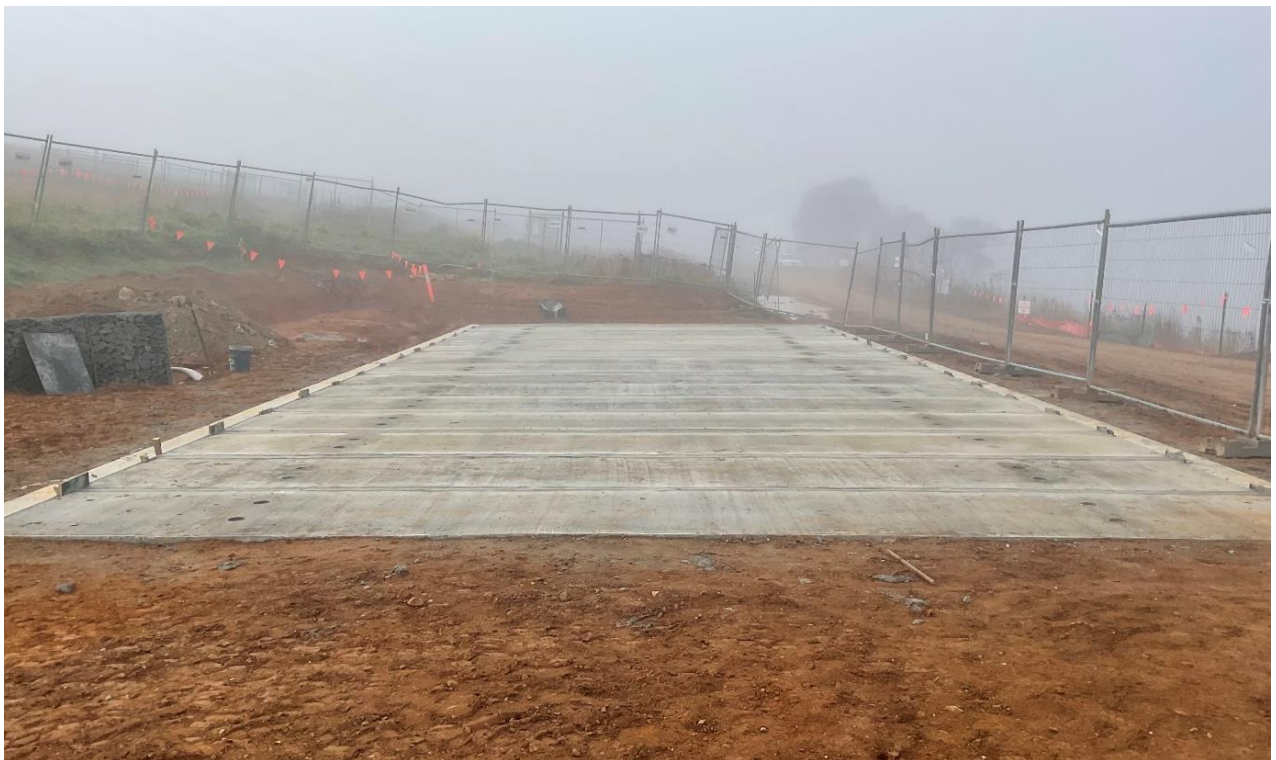
Figure 5.8.8 Bridging slab over asset
