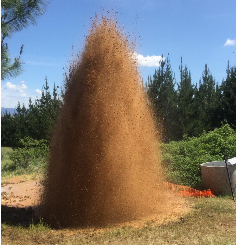
Figure 1.3.1 Burst DN600 water main and damage to the surrounding
