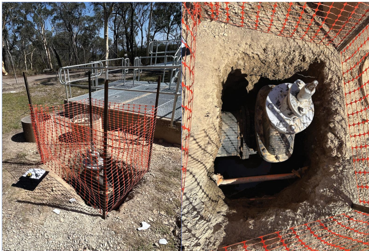
Figure 4.2.3 Hydrovac potholed gate valve and telecommunication cable
