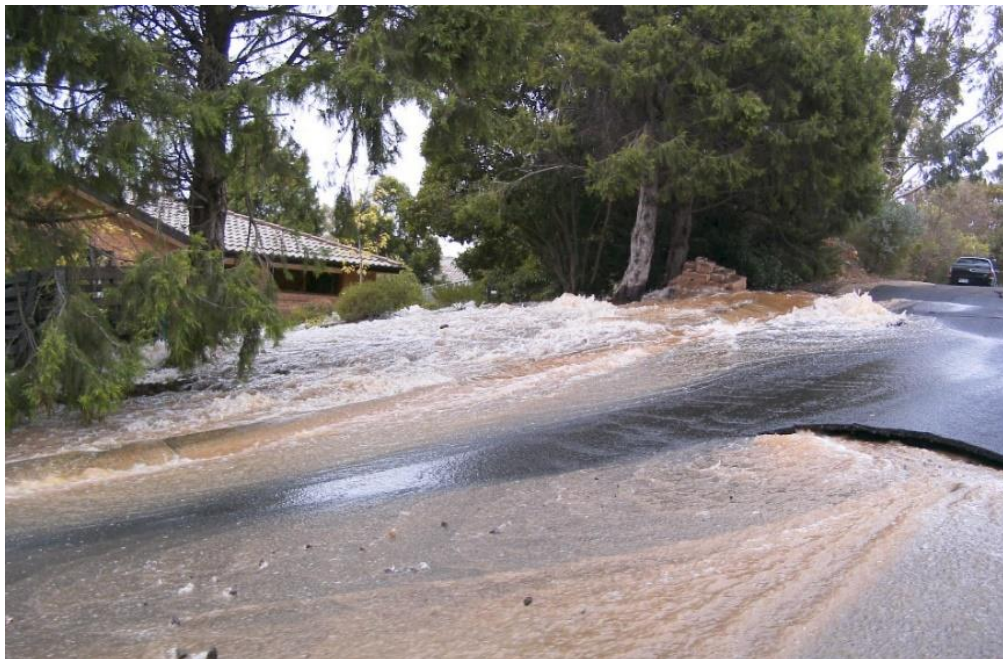
Figure 1.3.2 Damage to infrastructure and environment due to burst water main
