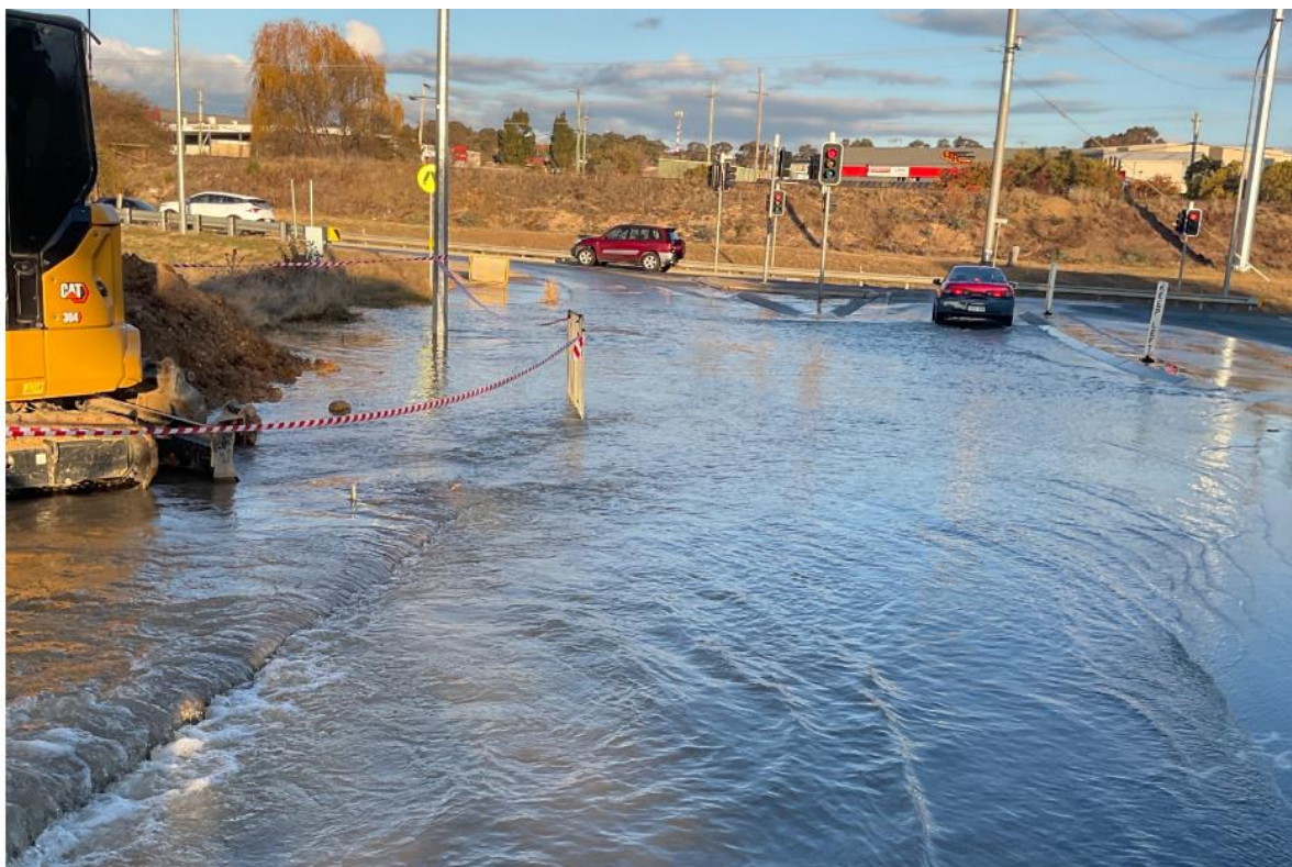
Figure 1.3.6 Impact of damaged water main on nearby infrastructure
