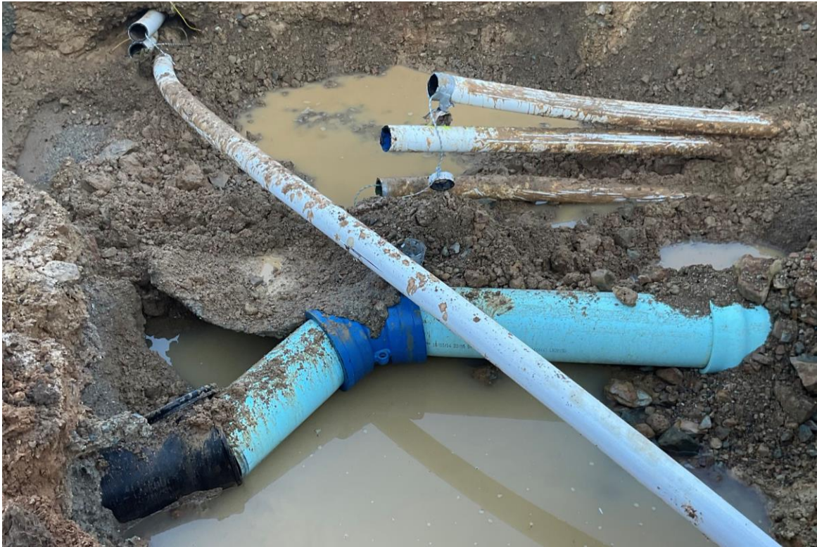
Figure 1.3.5 Service crossing resulting in damaged thrust block
