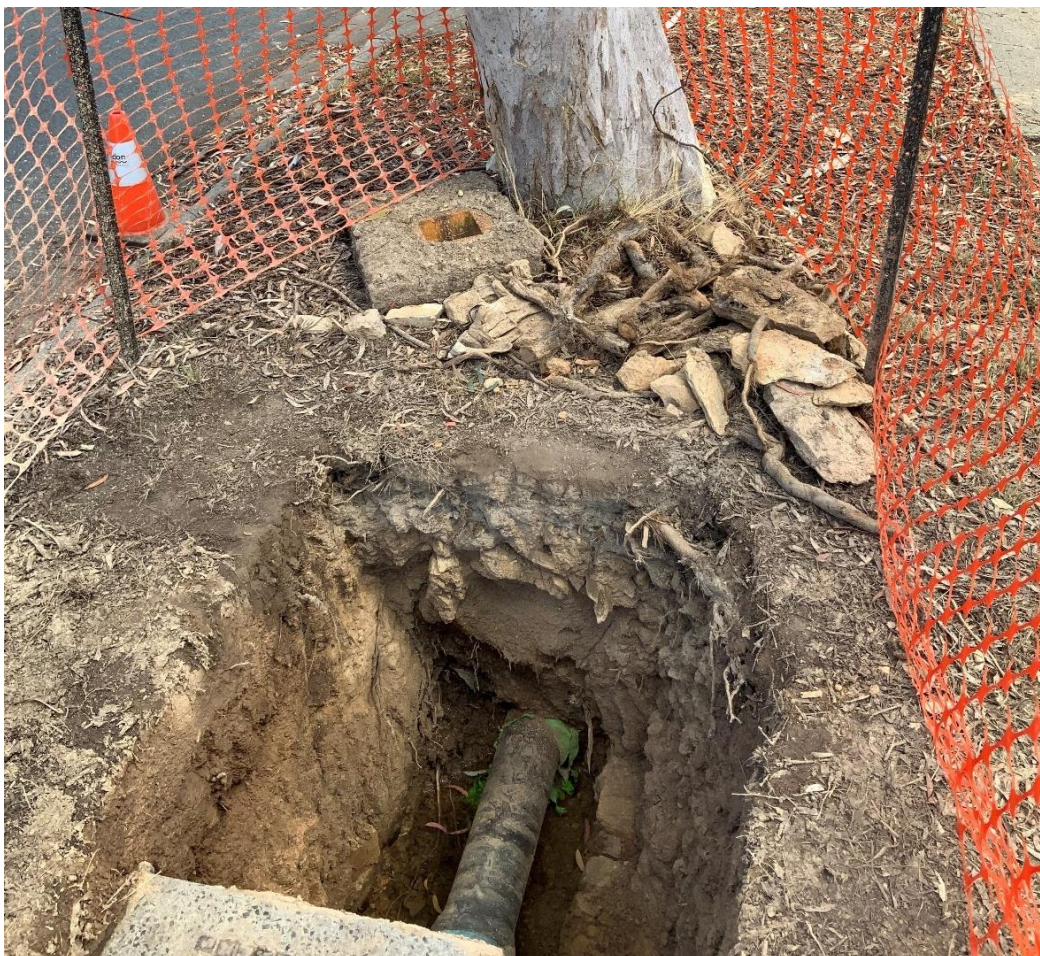
Figure 1.3.4 Tree roots impeding access to water main
