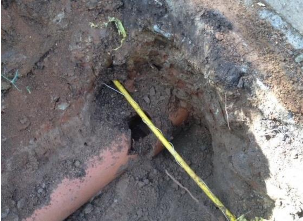
Figure 1.3.3 Damaged sewer main caused by horizontal directional drilling
