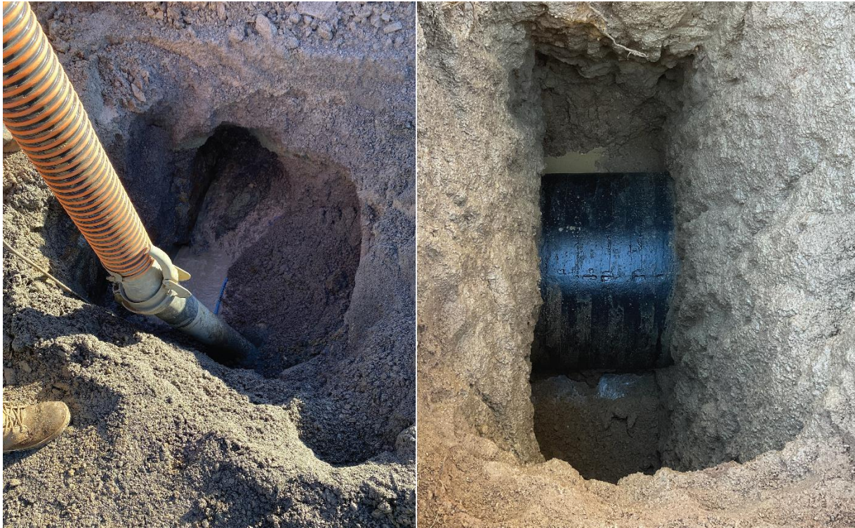
Figure 4.2.2 Hydrovac potholed water main
