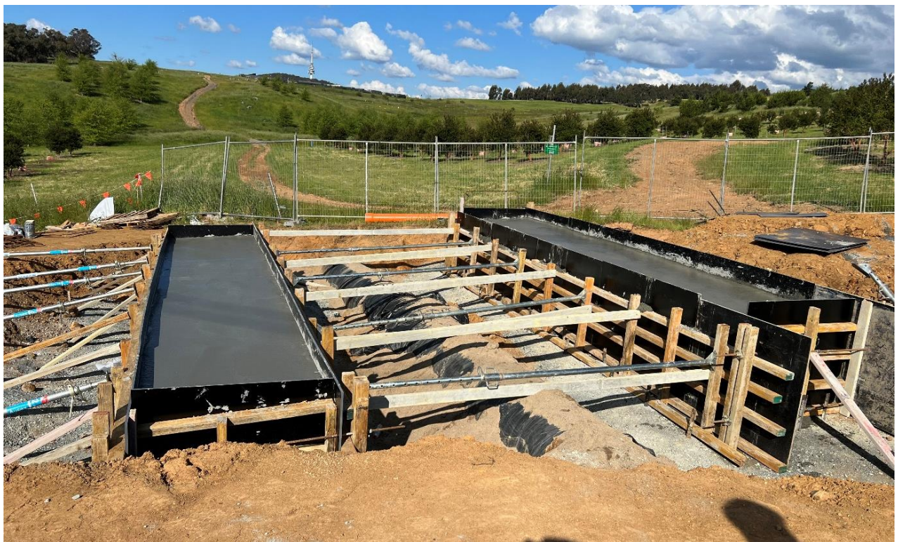
Figure 5.8.6 Bridging slab (under construction)
