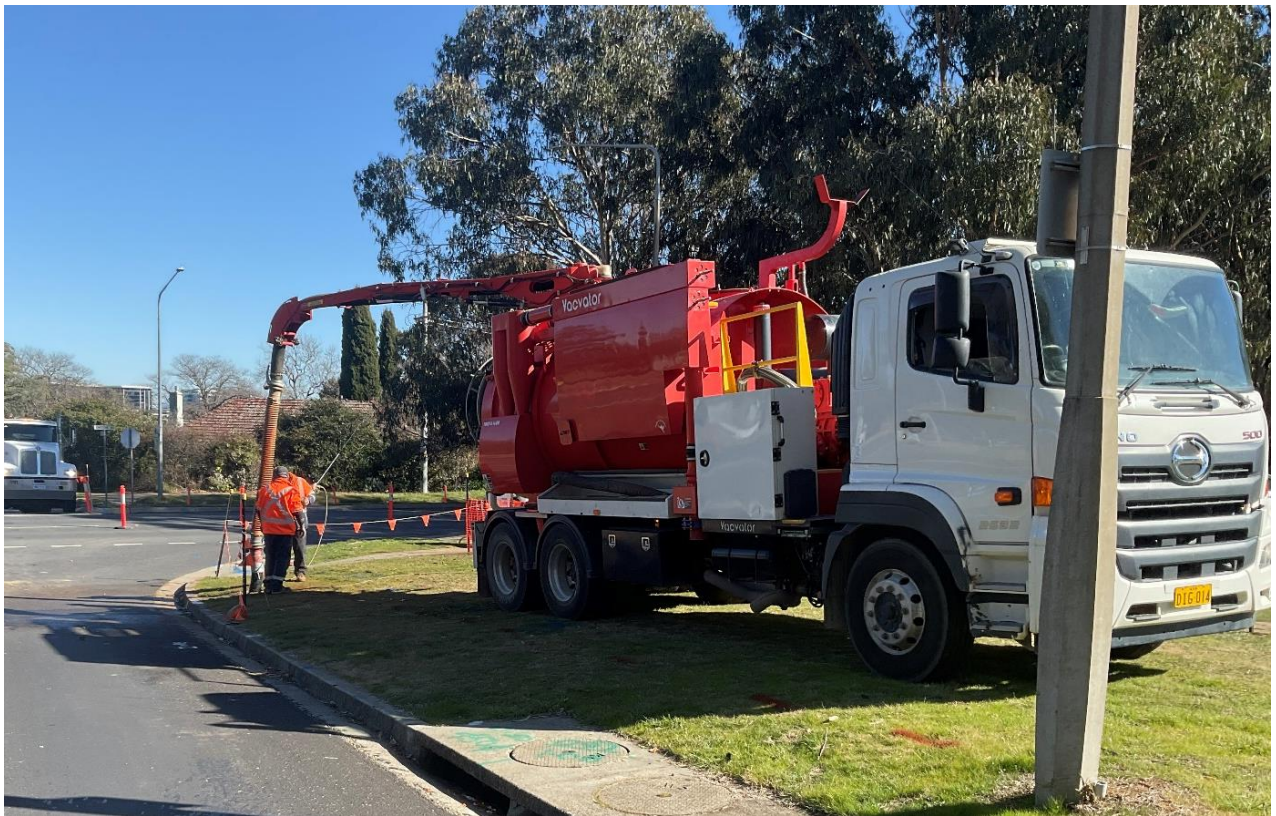
Figure 4.2.1 Hydrovac potholing in progress
