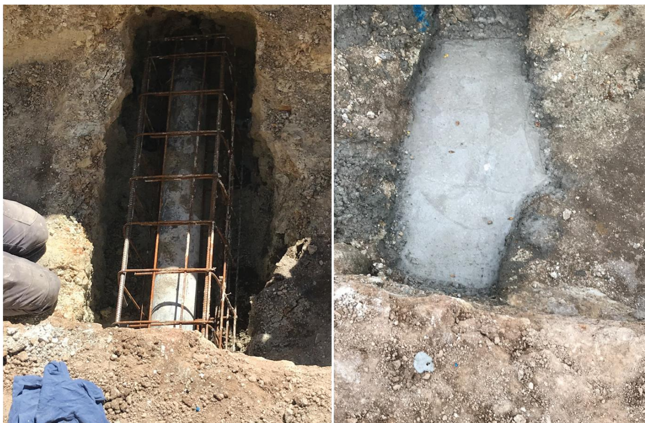
Figure 5.8.4 Concrete encased asset
