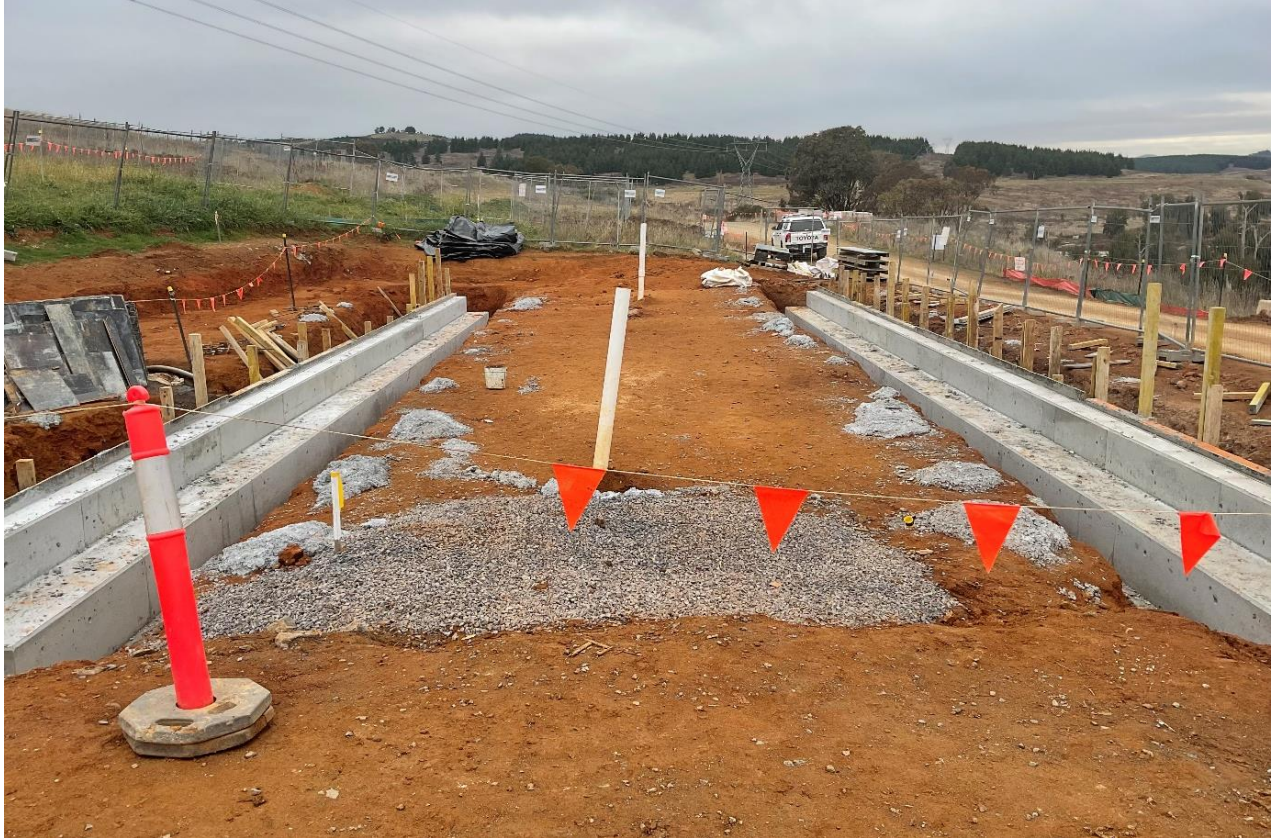
Figure 5.8.7 Bridging slab (under construction)
