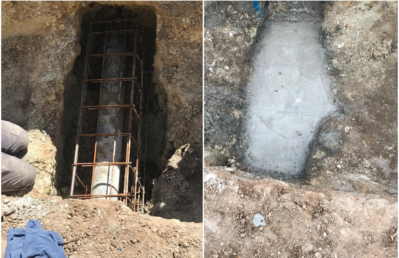
Figure 5.8.4 Concrete encased asset
