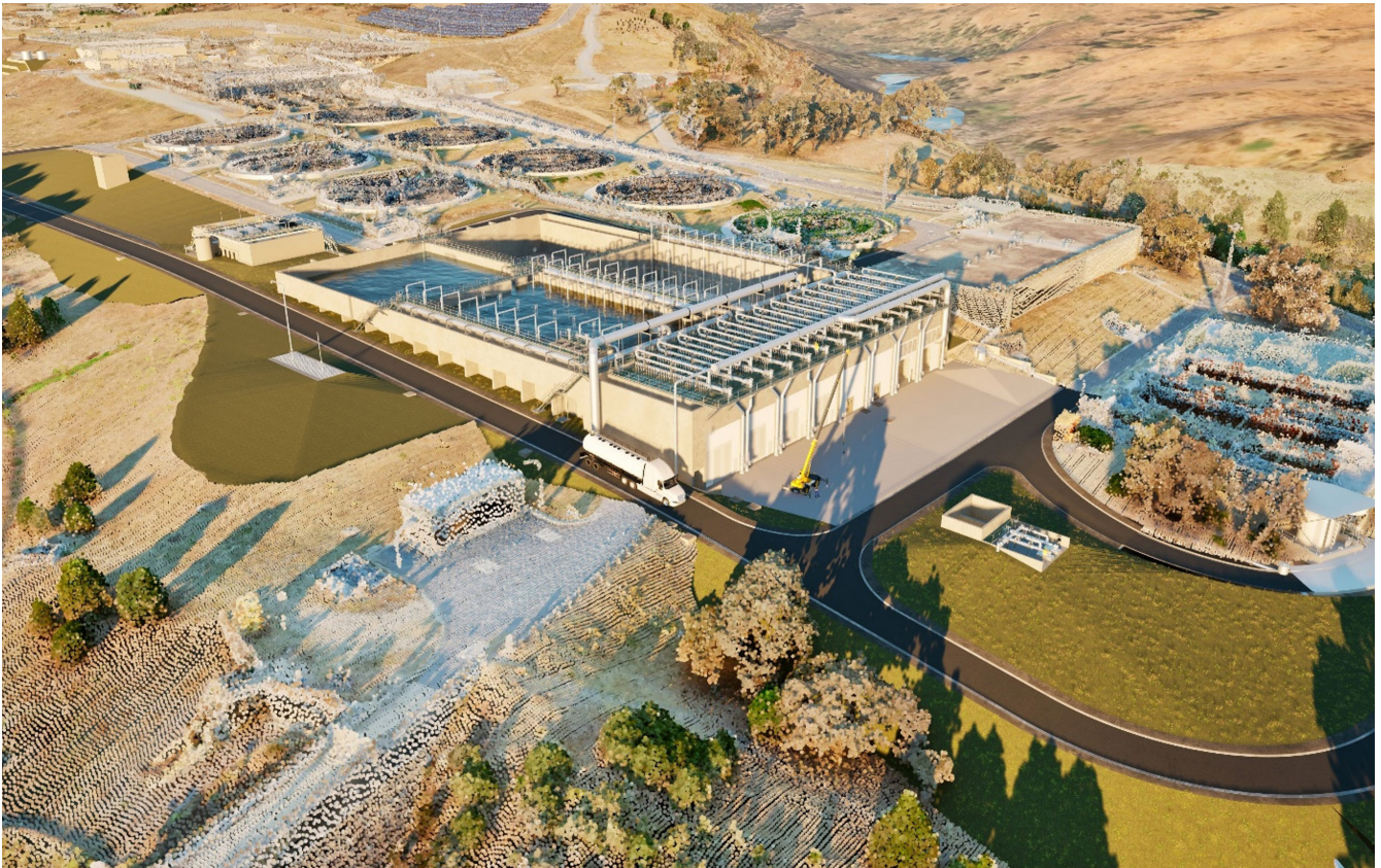
An artist impression of LMWQCC after the completion of the bioreactor project
