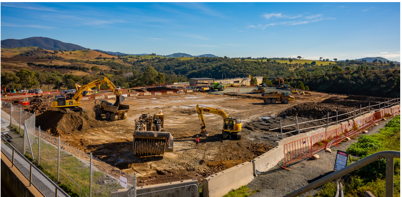
The excavation zone where our surface miner has cleared space for the new bioreactor.
