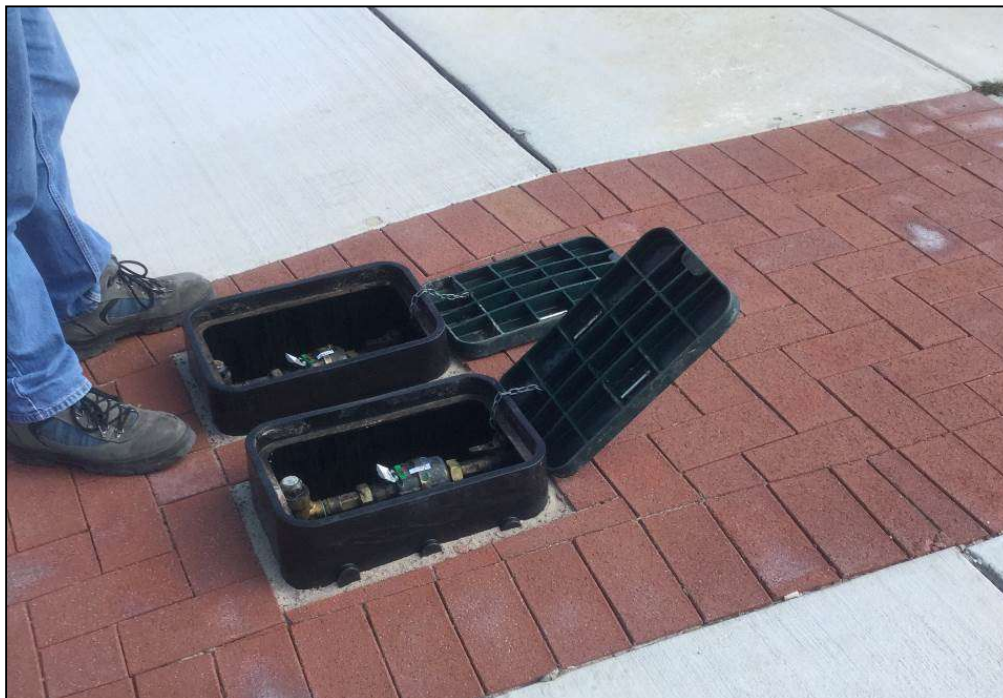
Figure Appendix A3 Failed DN20 Water Meter Installation (Water meter and meter box too high)
