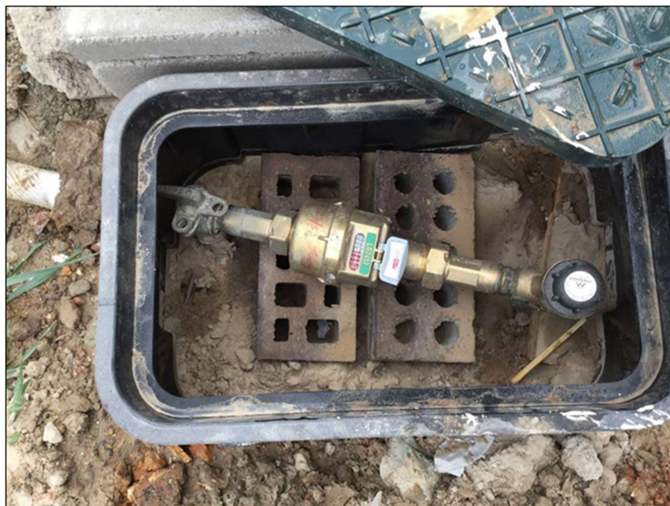
Figure Appendix A2 Failed DN20 Water Meter Installation (not centred; reduced valve clearance in box)
