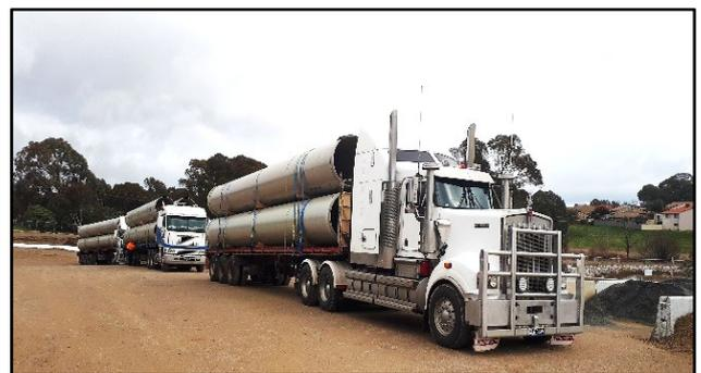
*1.8m sewer pipes arriving to the primary compound by truck ready for unloading and installing*
