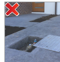
In driveway (unapproved)
